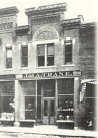
Trane Storefront La Crosse, Wisconsin 1891
